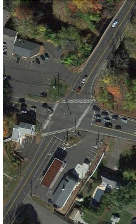
Intersection of Routes 68 and 150, where turning lane improvements should reduce congestion and accidents
